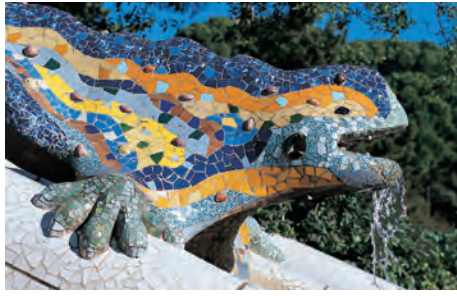
The mouth of the dragon in the entrance staircase of the Park Güell is the spout of the waters collected in the tank under the columned room
